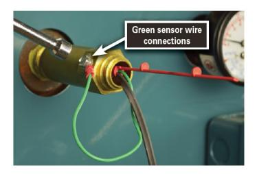
The inside of the well must be dry before installing sensor. Moisture in the well could lead to premature failure.
